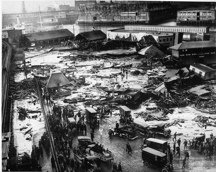
Figure 1. Aftermath of molasses tank failure
